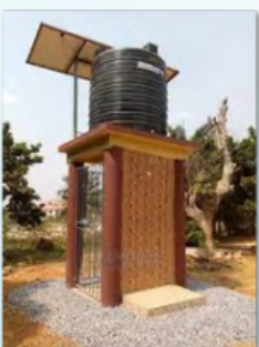
Example of a Solar Pump Borehole
